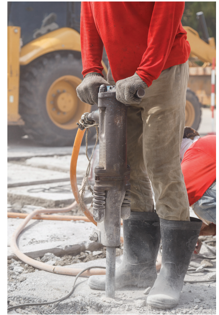
Figure 1.2 This kind of drilling can cause vibration white finger, and can also damage your hearing if the proper precautions aren't taken.
