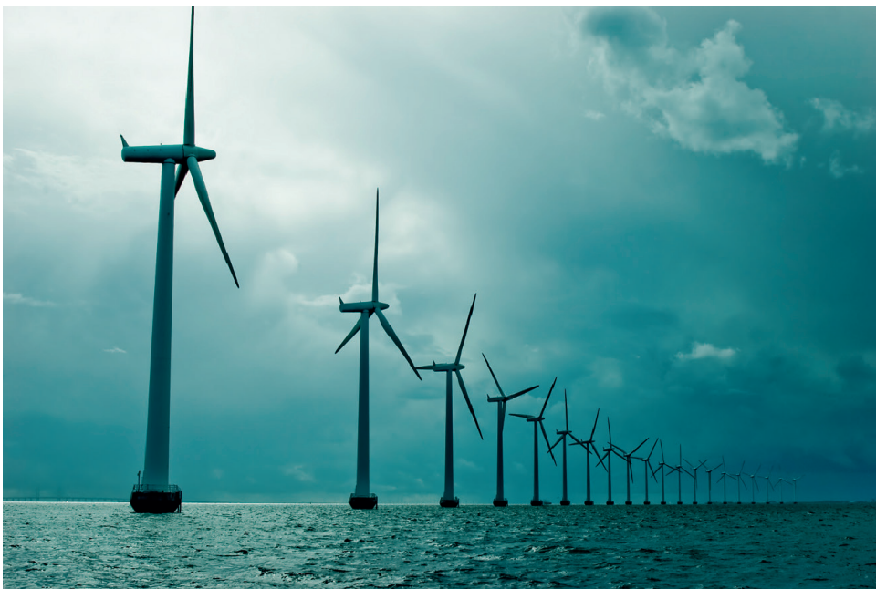
Figure 1.13 Offshore wind farm energy generators.
