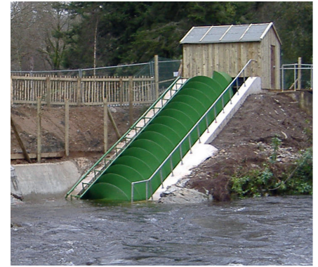
Figure 1.16 An example of an Archimedian Screw at the River Dart country park, Devon. Credit: WRE Limited.
